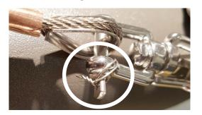
Slide the choked end of the lanyard back along the pole arm away from lantern until there is no slack! Strap the lanyard to the pole arm in 2 positions using cable ties! If not supplied, please ensure that UV resistant cable ties are used!
